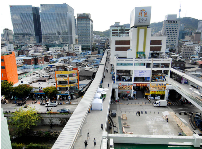
The third-floor decks stretch the entire length of the arcade buildings, flanking either side.
