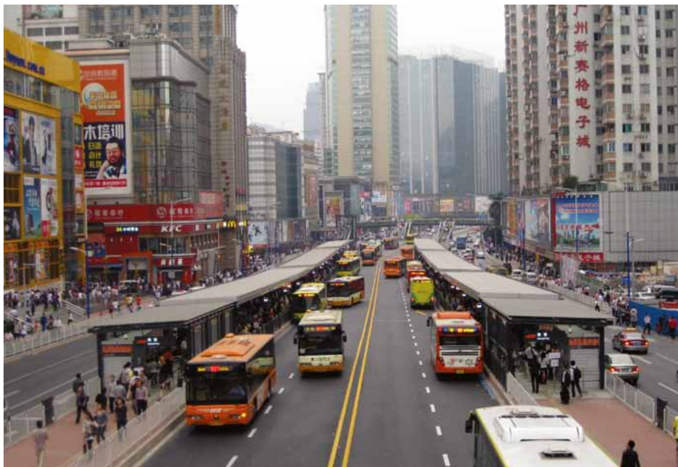
The Guangzhou Bus Rapid Transit system.
